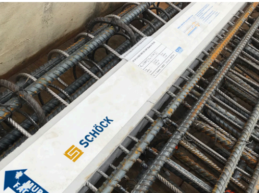
Isokorb® concrete-to-concrete connections for exposed slab edges
