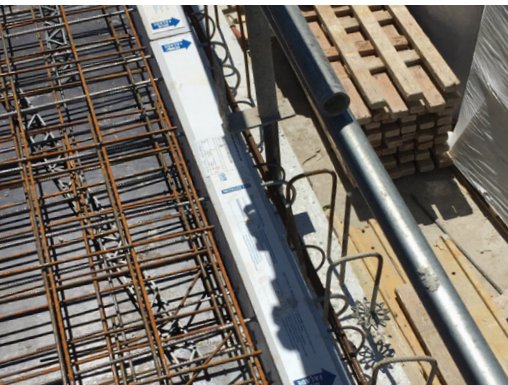
Isokorb® concrete-to-concrete connections for interior insulated walls
