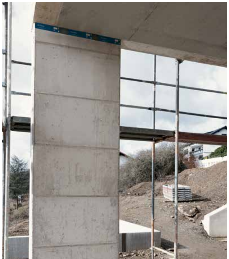
Sconnex® creates slim wall profiles with an exposed concrete finish and lastingly eradicates thermal bridging.
