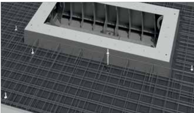
4. Insert Schöck Isolink® type C-SH into the predrilled thermal insulation layer
