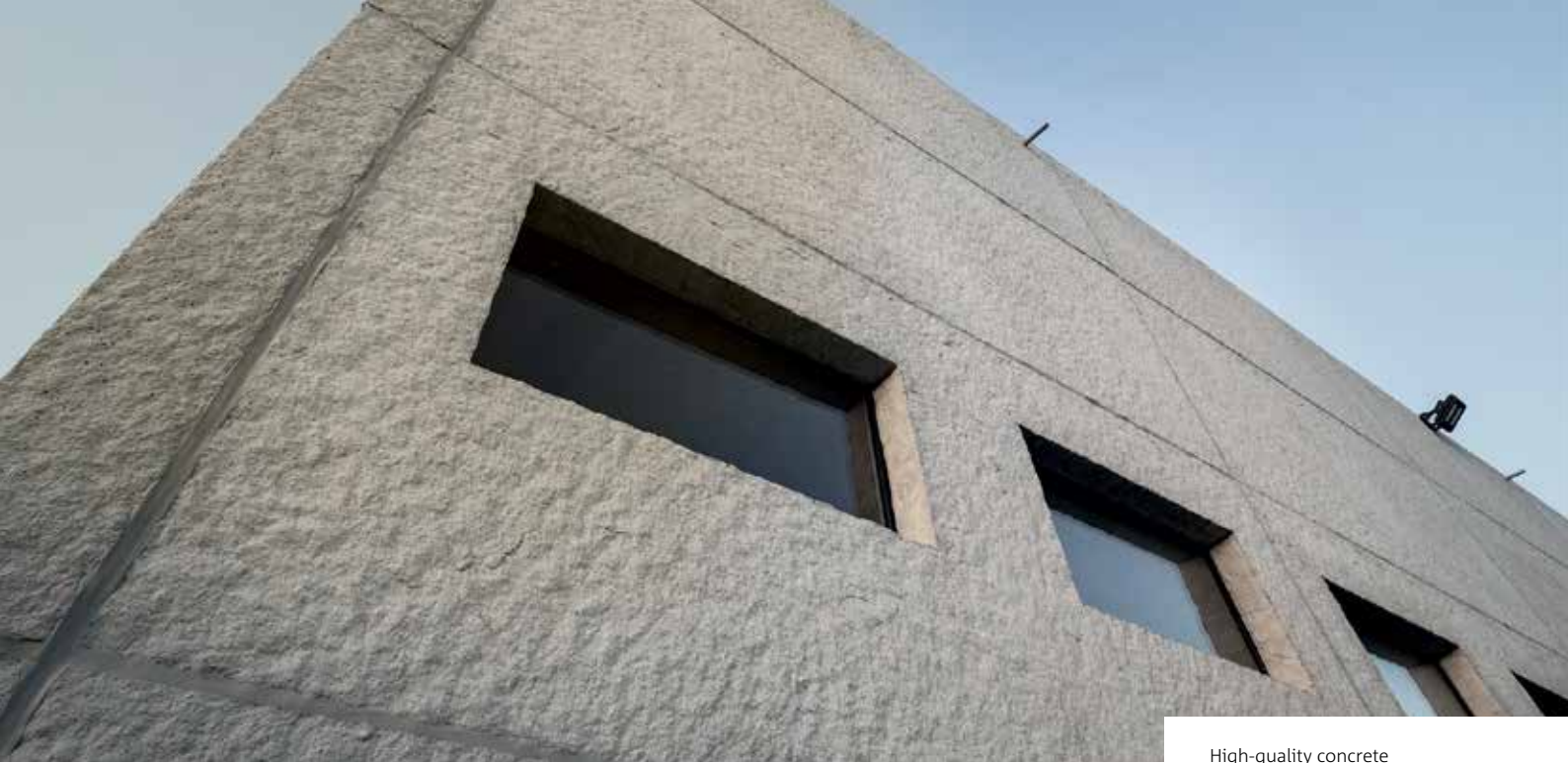
High-quality concrete façade in natural stone look for the Marcus Riedelsheimer GmbH industrial building
