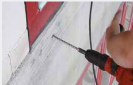
Links: Bohrlochschablone anbringen
